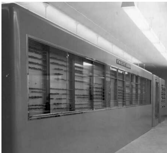
The system installed at ASEA
